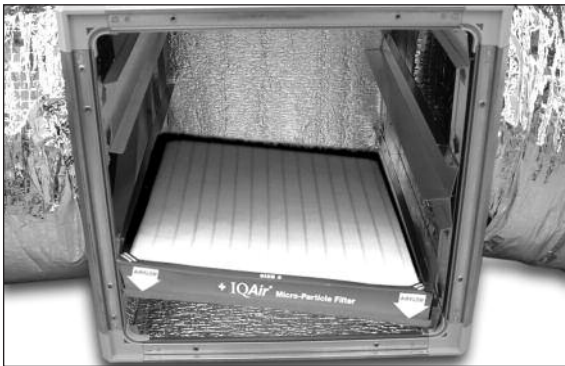
5. Insert new filters starting from the bottom.
