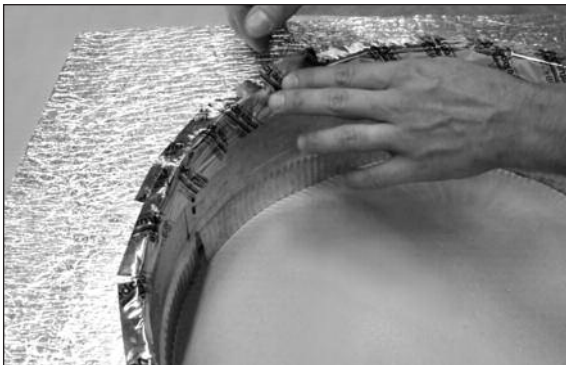
11. Stick the tape tightly to the insulation.
