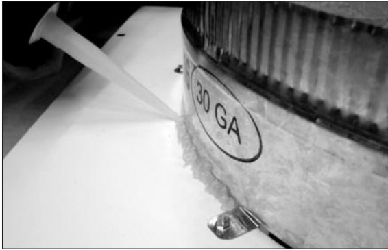
9. Seal the gap between the collar and the panel and wait till it has dried.
